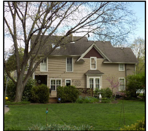
2015 – west side of home
