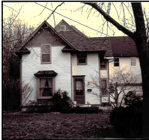
1999 – south side of home / South Street
